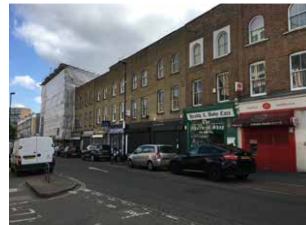
Above: No.s 186- 214 (Even) Attractive and largely uniform, three storey Victorian terrace with sash windows and butterfly roof.
