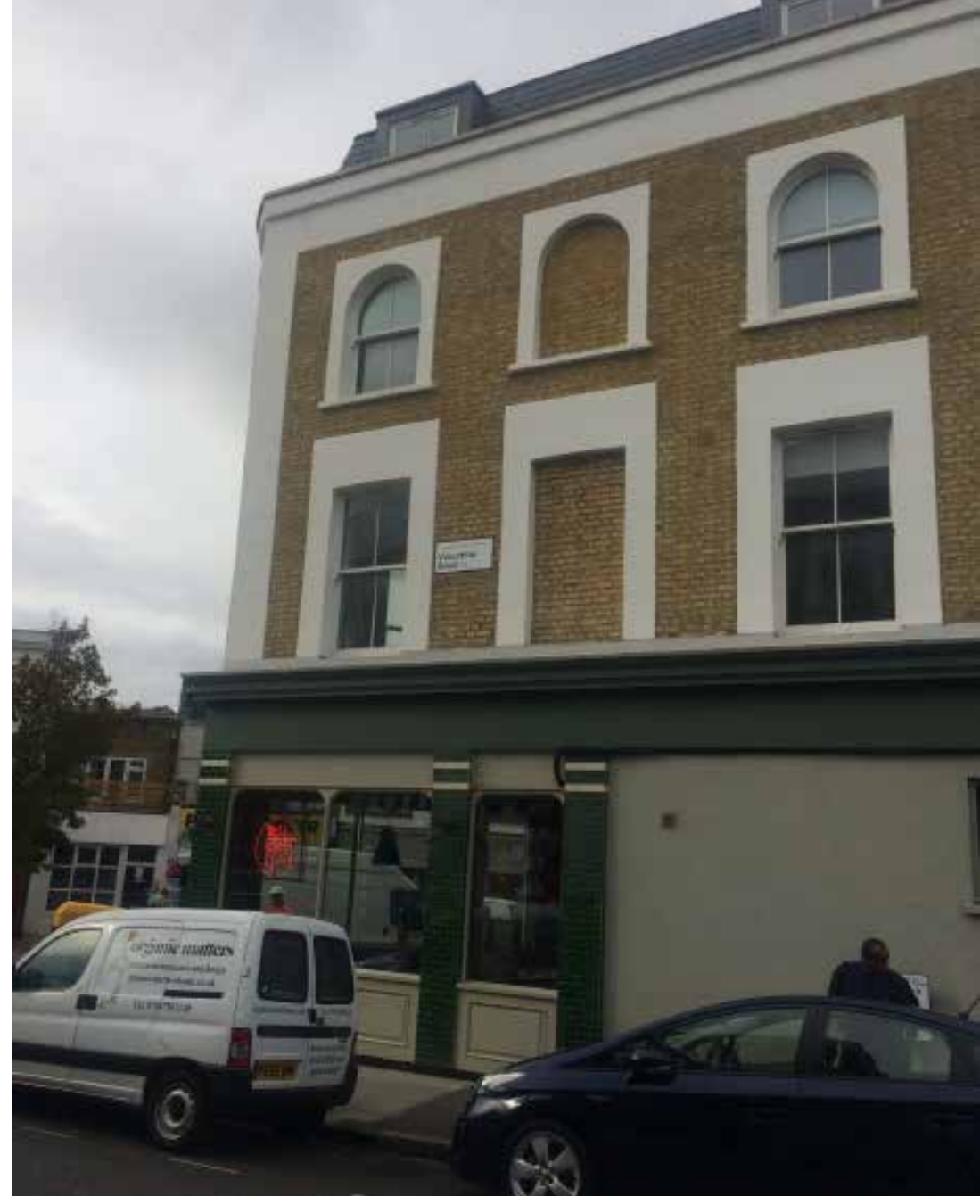
Former pub at corner of Well Street and Valentine Road
