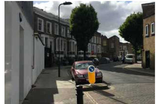
Above: No.s 36- 42 (All) Part 2/part 3 storey terrace with projecting front bay and unbroken cornice detail.
