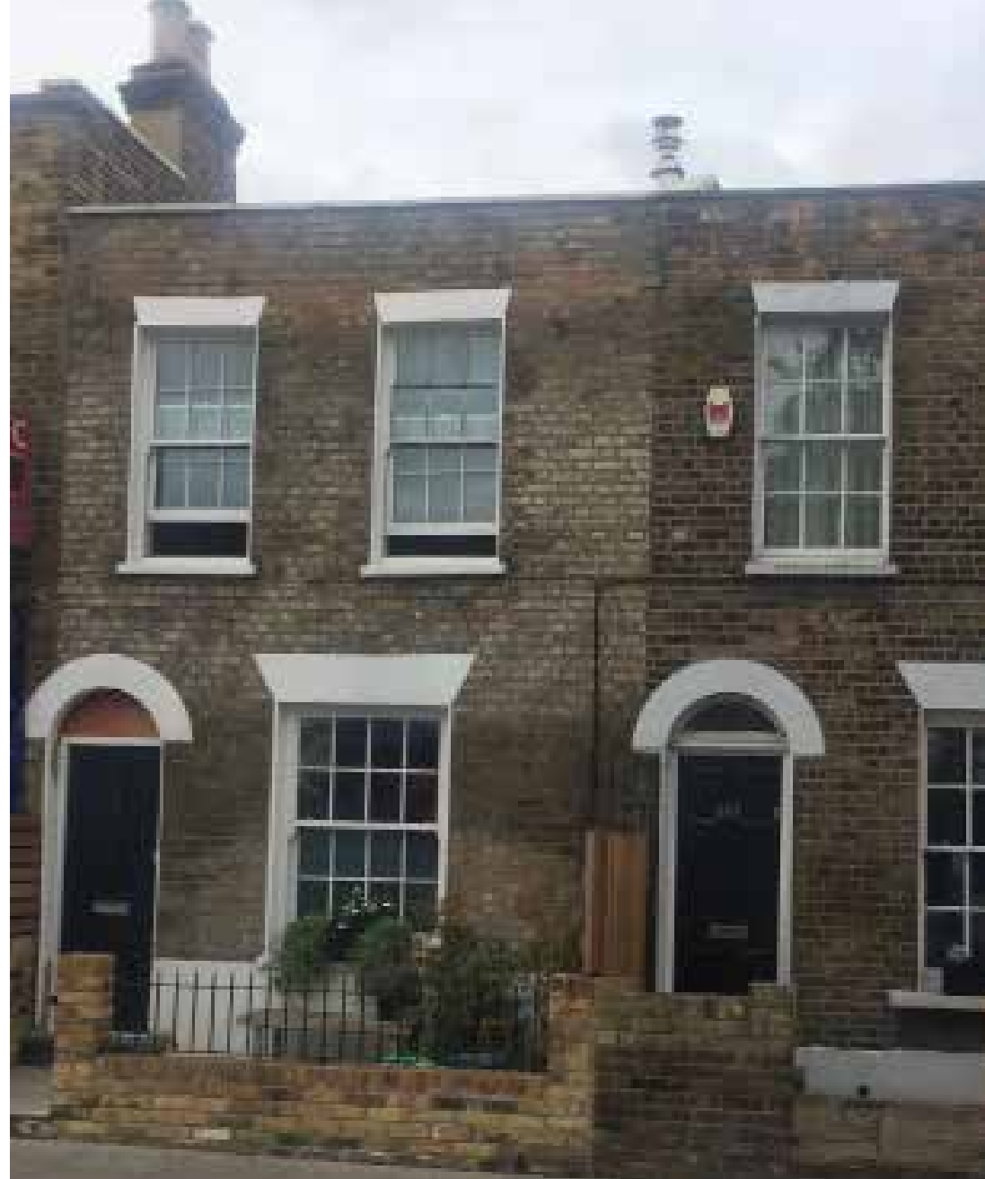
Early 19th century terrace, Well Street
