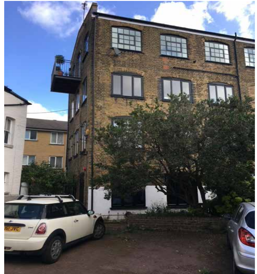
Former warehouse, Millborne Street
