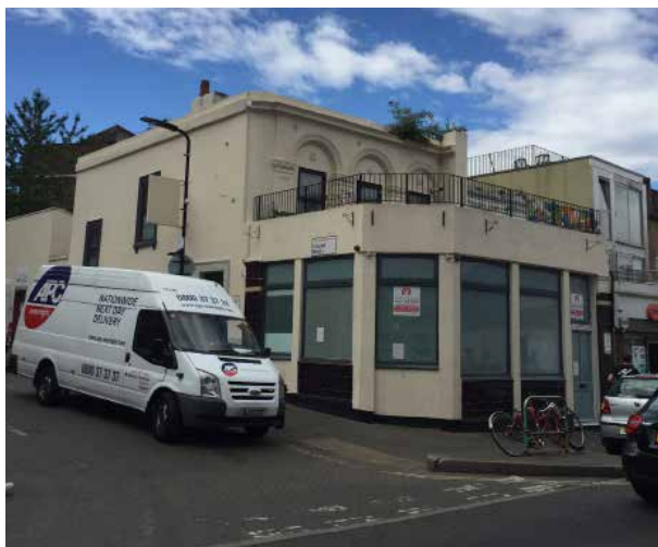
Below: No. 237 Former Brunswick Arms PH Former Victorian pub now in use as a mosque. Locally listed.
