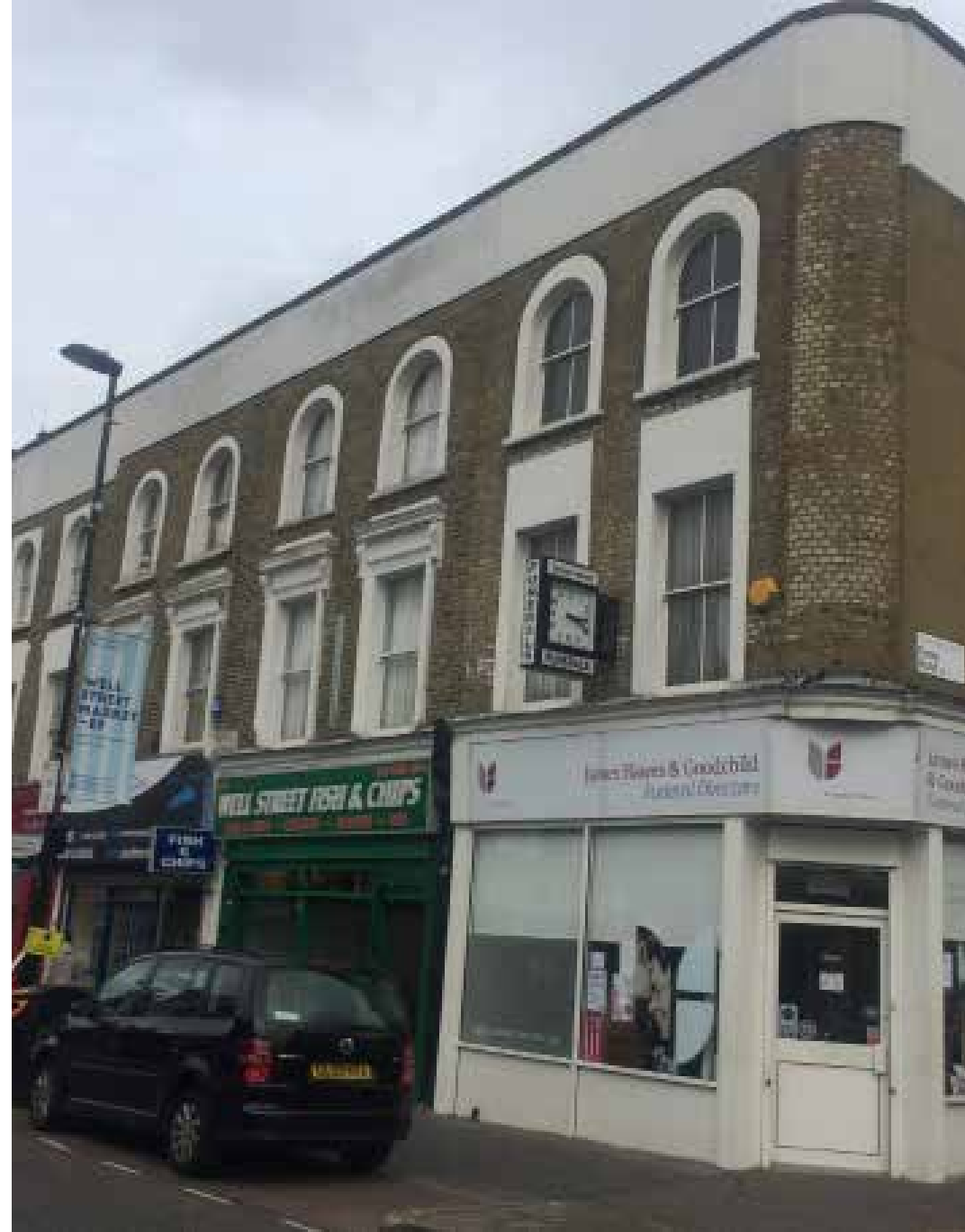
Terrace on Well Street
