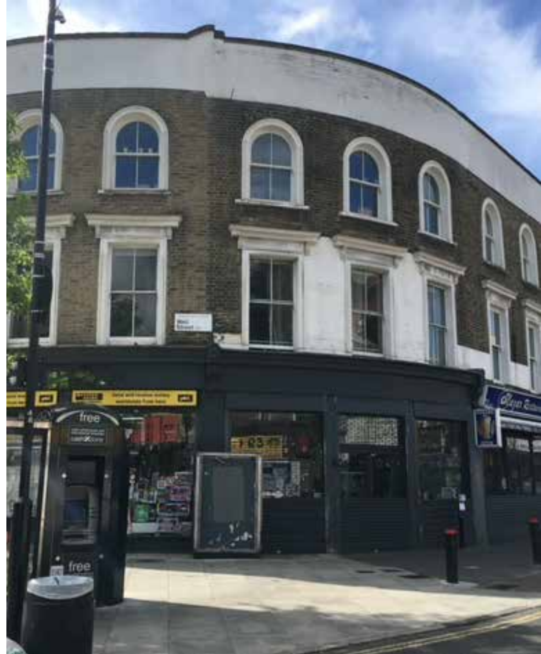
Curved terrace on Well Street
